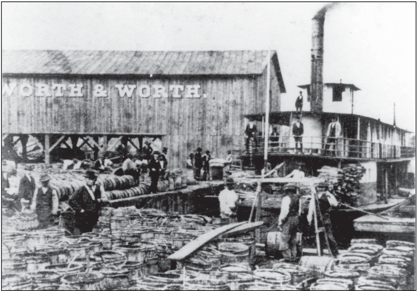
Figure 6. McEachern's Wharf, Wilmington, NC.
