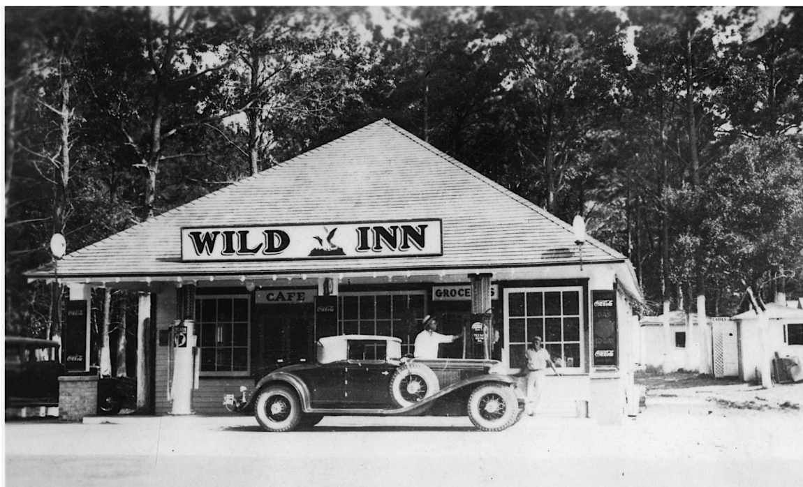
Figure 9. Built in the winter of 1931 as part of the initial development of Dare County, the Wild Duck Inn included a restaurant, a filling station and a campground (Photo courtesy of the Outer Banks History Center).
