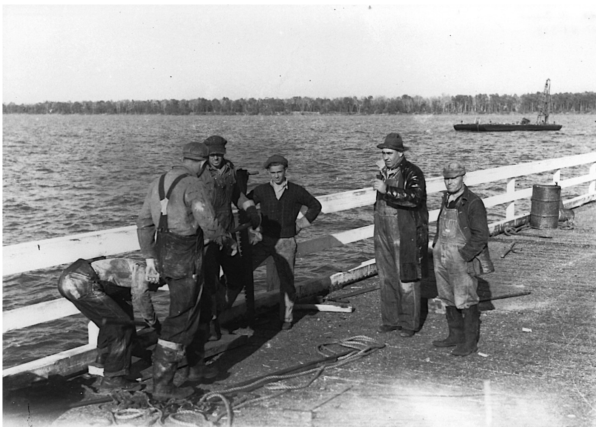
Figure 5. Employees of the W. L. Jones Construction Company take a break from laying the deck of the Wright Memorial Bridge (Photo courtesy of The Outer Banks History Center, Ben Dixon MacNeil Collection).
