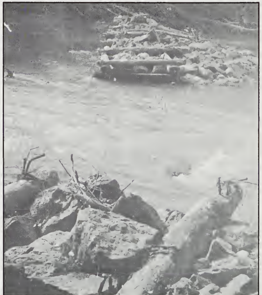
Wing dams constructed with log cribs by S.T. Abert, c. 1885, at Slink Shoal on the Dan River (Lindley Butler)
