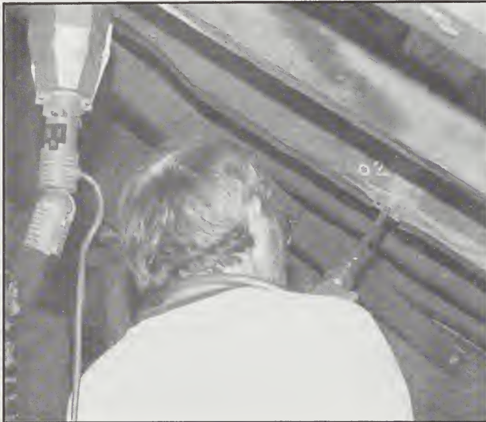
Taking a core boring from the Cupola House.
